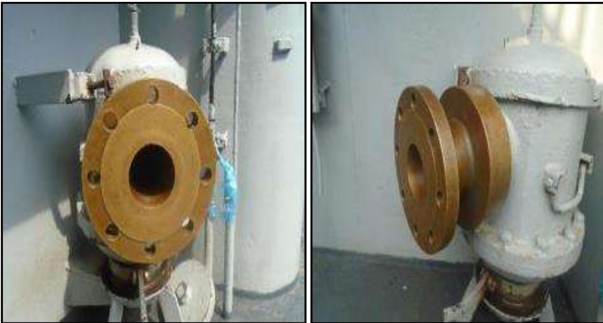
Picture 6 – Fuel Coupling (Type A): Front View (Left) and Side View (Right)
